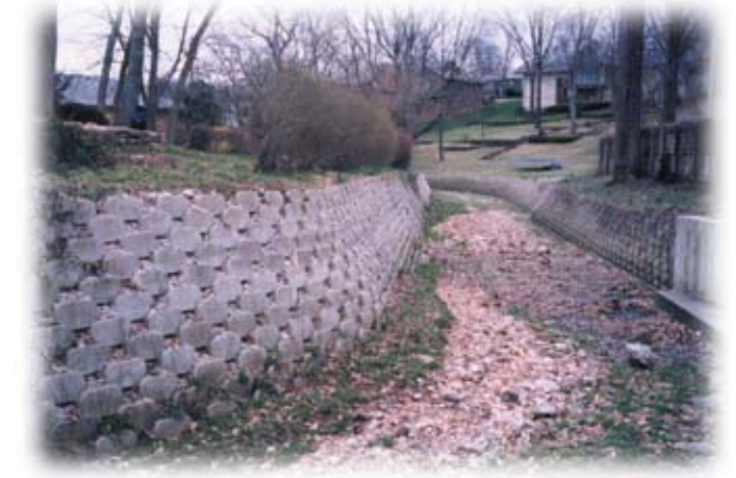
Residential creek bank gravity wall, after 10 years in place.
