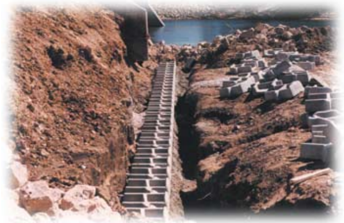
Bridge approach protection.
