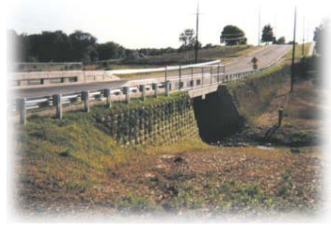
Scour protection for bridge over creek.
